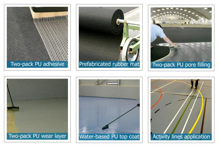
All materials used in the formulation and installation of these products are environmentally friendly, utilising recycled rubber for the prefabricated mat together with solvent-free and water-based polyurethane technology.
