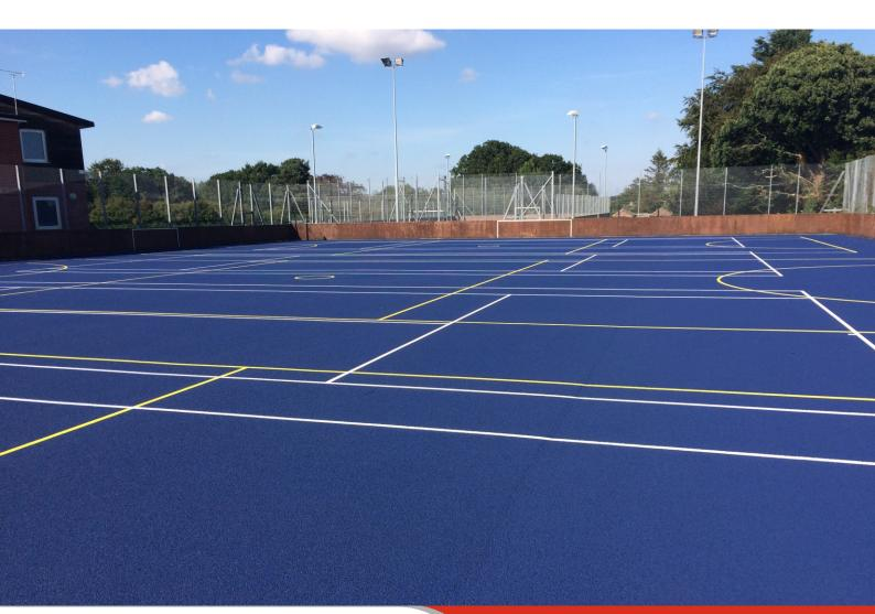
Sports-Cote<sup>™</sup> Sports-Line Acrylic is applied using airless spray unit, brush or medium pile roller
